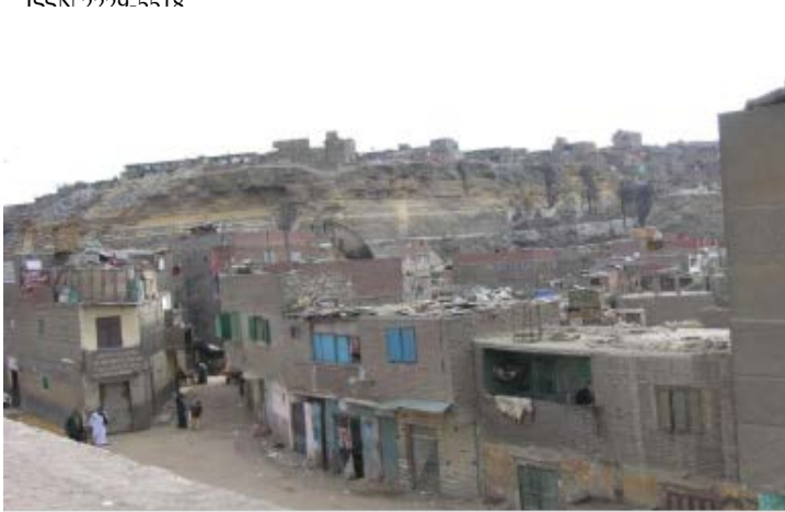
Fig. 2 Informal Housing in Ezbet Bekhit
